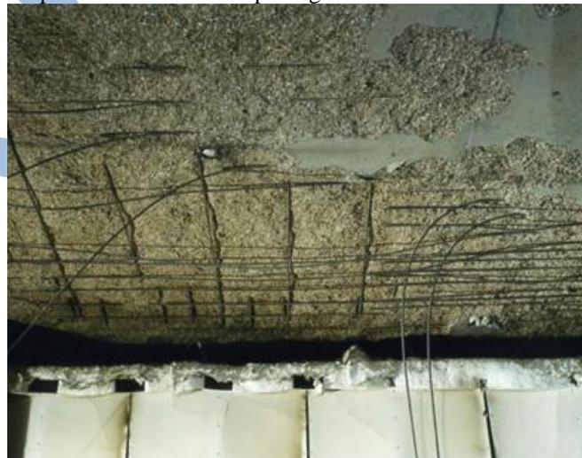
Figure 1 (Showing spalling of Concrete)
